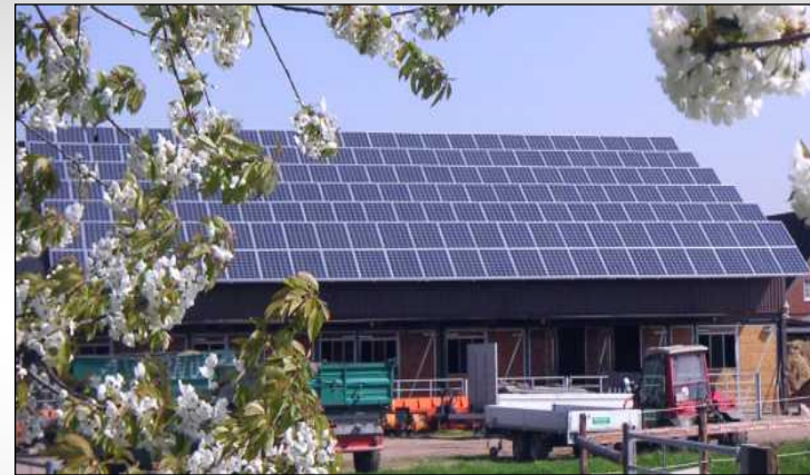
50kW Hamburg, Neuenfelde
